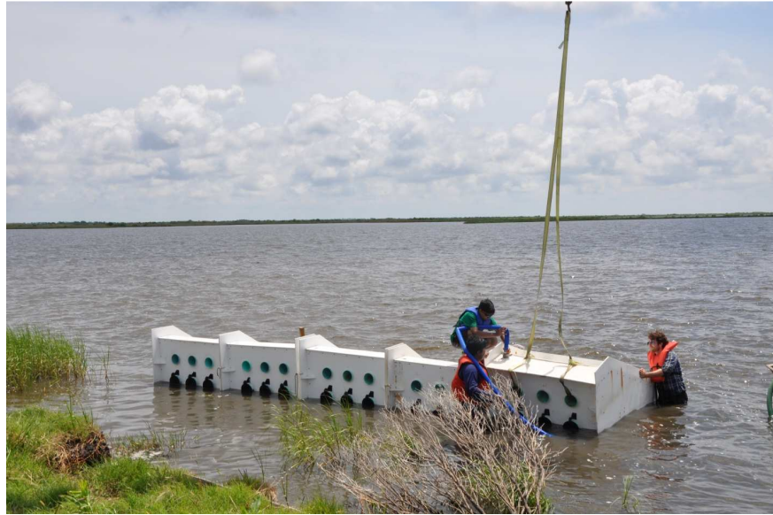
Figure 13: WSSC Units Being Filled with Water and Placed at Site
