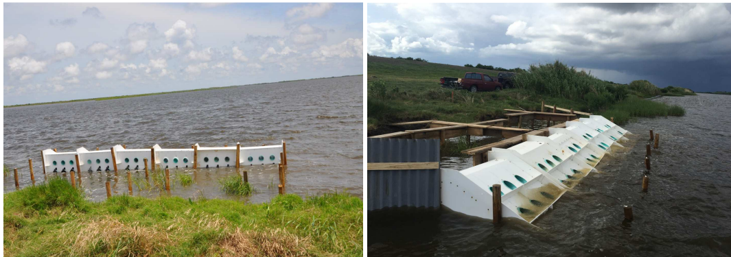
Figure 14: WSSC Units after Construction
