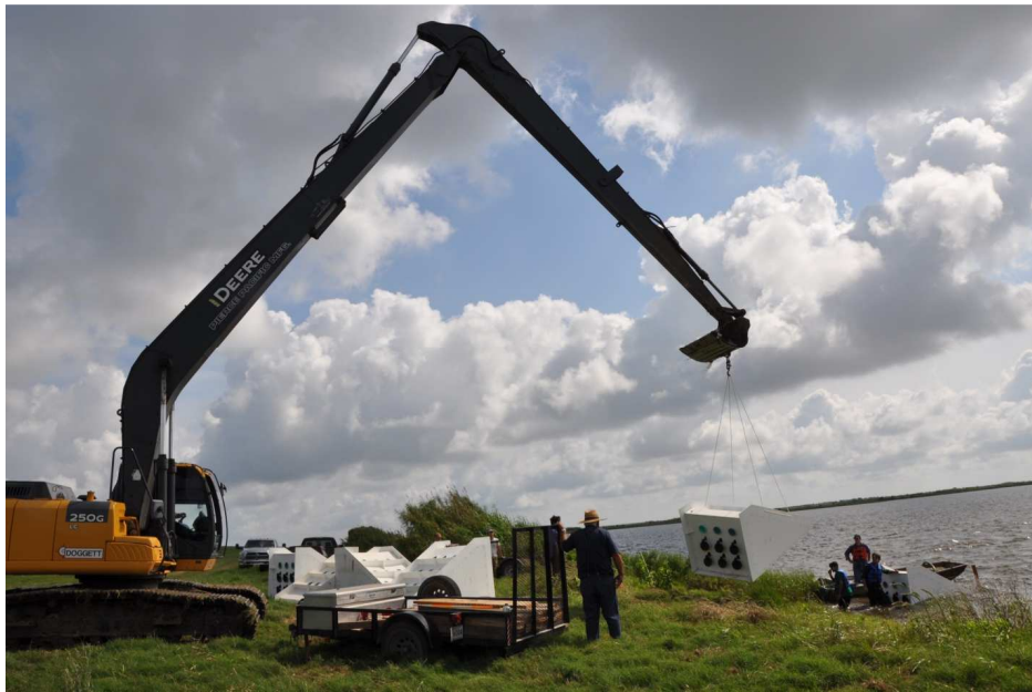
Figure 12: WSSC Units Being Installed in the Site
