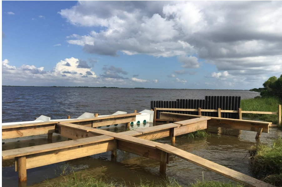
Figure 15: WSSC Units with Wooden Bridge for Walking
